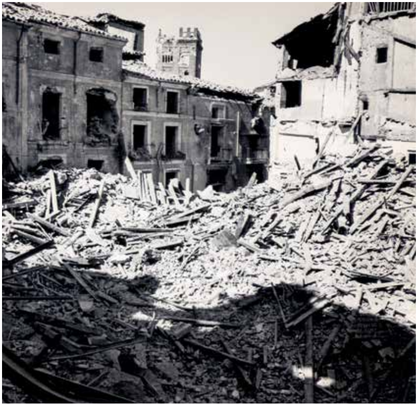
Teruel. Banco de España. Building destroyed during the Civil War. c. December 1937-February 1938. Photograph: Marquis of Santa María del Villar. Gelatin silver.
