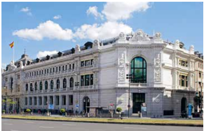
Above and center: Madrid. Banco de España. Competition of preliminary proposals for the closure of the building on the streets of Alcalá and Marqués de Cubas. Projects by Corrales and Molezún and Moneo. 1979. Photographs: Altair Photo. Chromogenic prints. Below: Madrid. Banco de España. Extension of the building on the streets of Alcalá and Marqués de Cubas. 2006. Digital image.
